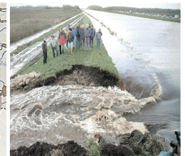
Release of canal breaking a dike. The Netherlands
