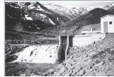
Micro Hydro Facility in King Cove Alaska(800kW)
