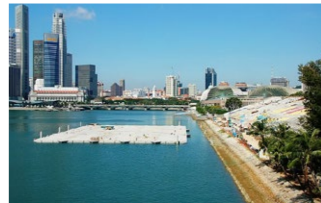
VLFS technology - Very large floating structure
