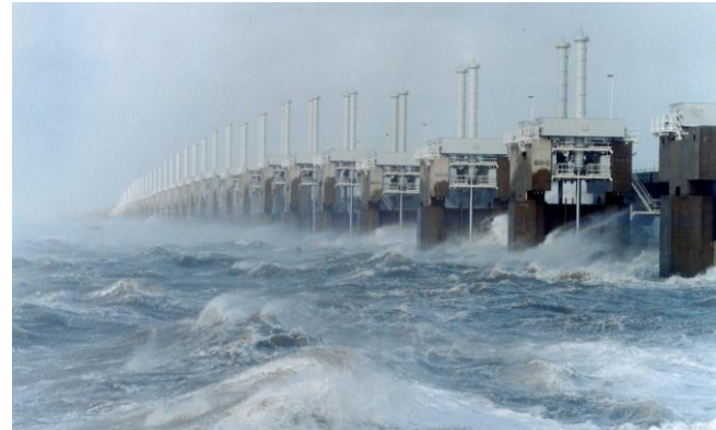
The Oosterschelde storm surge barrier, Netherlands
